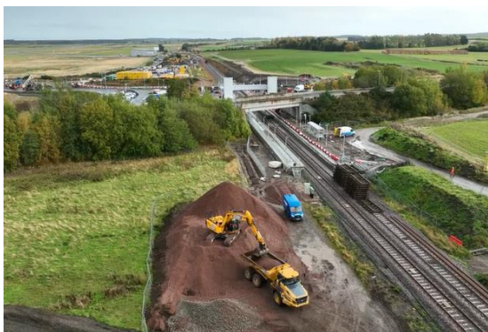
Picture 3: Inverness Airport Railway Station Oct 2022
