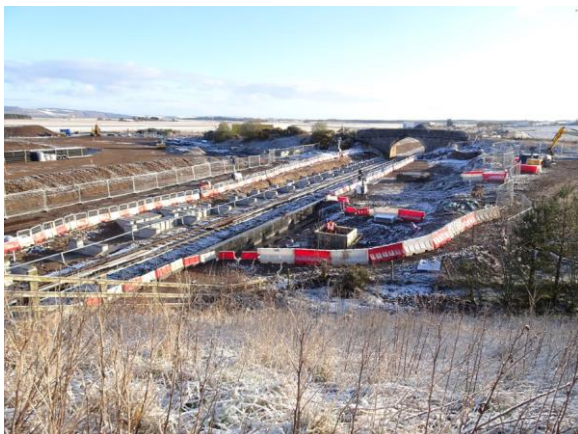
Picture 1: Inverness Airport Railway Station development
